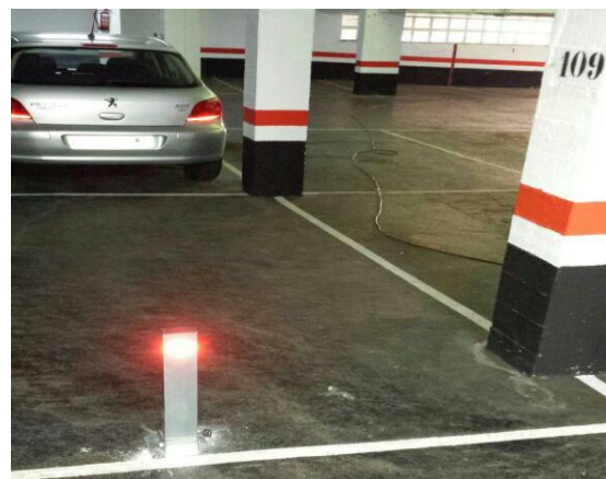
Installation in parking
